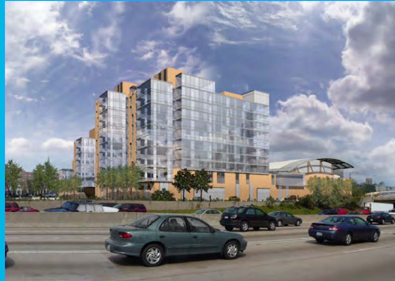
James J. Stukel Towers Residence Hall and UIC Forum, from Dan Ryan Expressway
